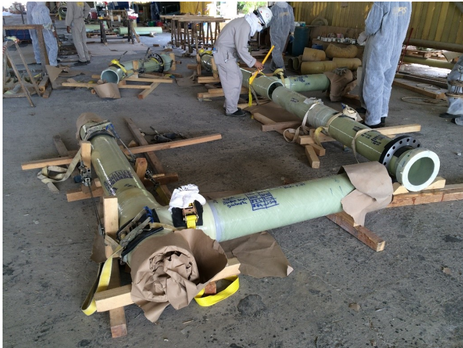
“Training in Oman, adhesive bonded joints, 2 crews making a spool”
