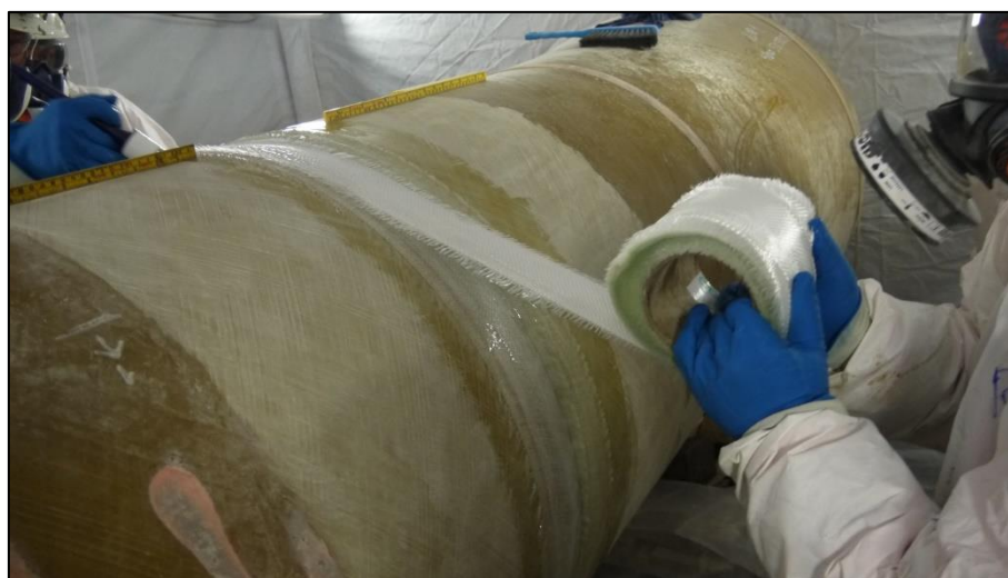
Figure 8: Applying fit laminate (Courtesy FPI).
