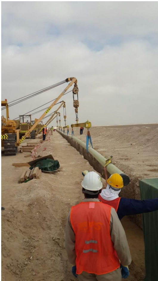
Figure 2: Field installation of buried GRP/ GRE piping in Oman (Courtesy Jishnu Narayanan Kutty).
