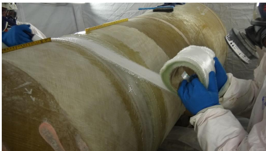
Figure 8: Applying fit laminate (Courtesy FPI).
