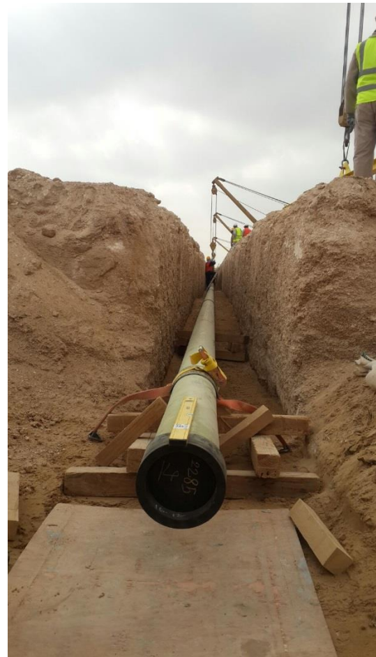
Figure 2: Field installation of buried GRP/ GRE piping in Oman (Courtesy Jishnu Narayanan Kutty).
