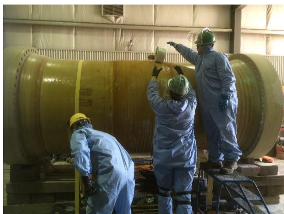
"laminating structural layer"
